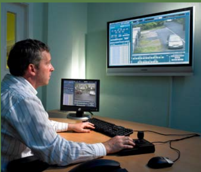
Purpose built control facility within the Town Hall at Colne including a WV-CU650 system controller
