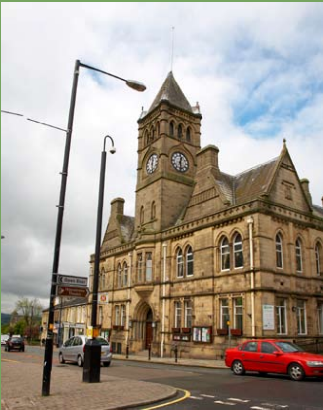
One of eight Panasonic WV-CW960 Weather Proof Super Dynamic III Colour Dome Cameras installed at Earby and Barnoldswick town centre
